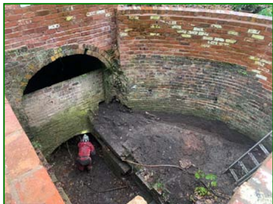
Vicky measuring distances in the main culvert.
