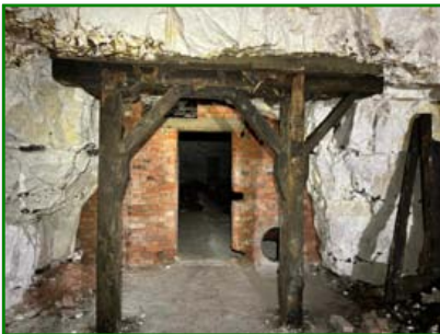
A former storage area. (Oliver Beard)
