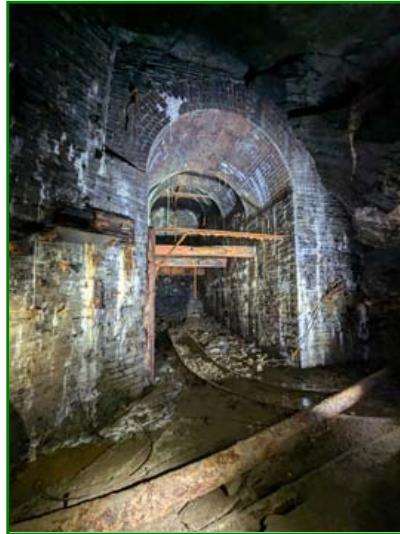
The brick built incline-head. (Keith Whiddon)
