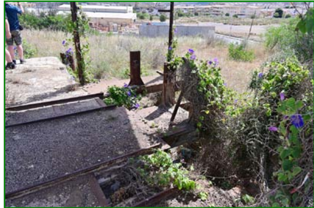
Tippler by the shaft of Mina Ocasión, Pozo Carmelo.
