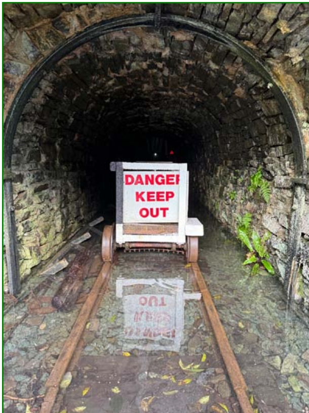
Flood water at the entrance up to the base of the truck. (Kelvin Lake)
