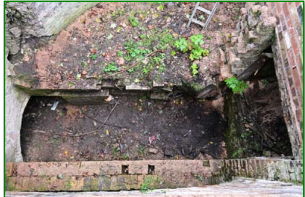
The pit with the long bolt top of picture, culvert to left.
