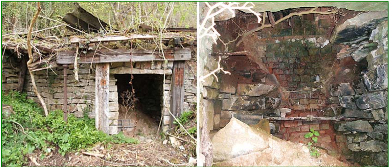
Figure 12: Lime kiln in Breakwell's quarry. Left: exterior; right: view through draw hole.
