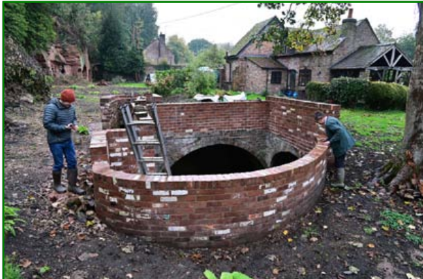
James and David by the new pit wall. (Kelvin Lake)
