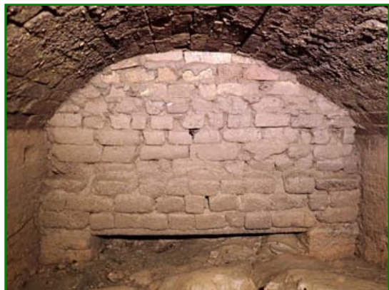
Culvert wall under the smithy.
