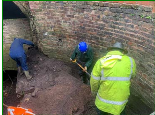
David, Steve & Andy digging in the pit.
