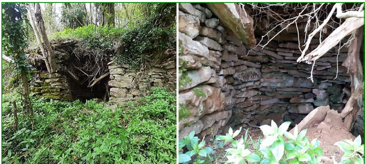
Figure 8: Lime kiln in Breakwell's quarry. Left: exterior; right: view through draw hole.
