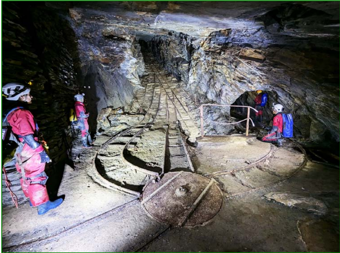
The elegant track layout at the head of an incline which enables wagons to access the incline by means of the small turntable in foreground. (Keith Whiddon)
