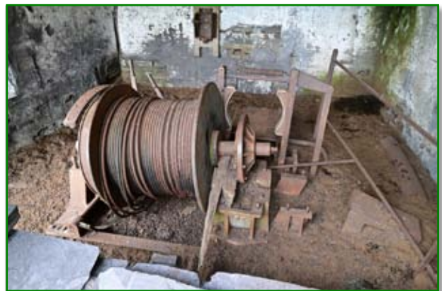
One of the electric haulage winches, Albion Level.
