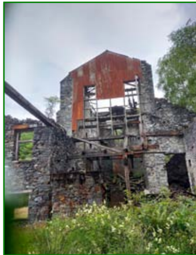
Klondyke mill. (Andy Wood)
