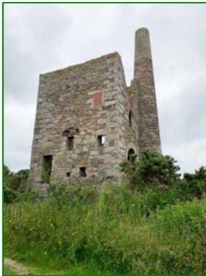
George's shaft 70" pumping engine house. (Gareth Rushton)
