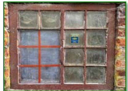
Nick's temporary repair.
