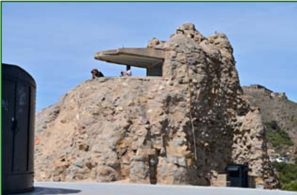
Fire direction control tower for gun No.2, with Atalayón Battery (349m above sea level) on hill behind.
