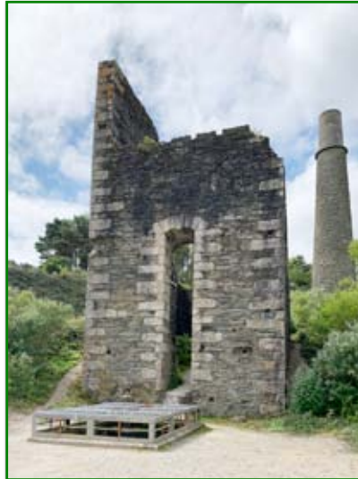
Taylor's 85" pumping engine house of Wheal Virgin. (Gareth Rushton)
