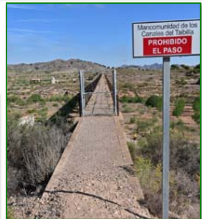
The enclosed top of the aqueduct.
