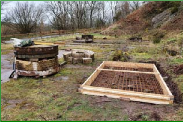
Preparing the display slab, 19 th March 2020. (Andy Wood)
