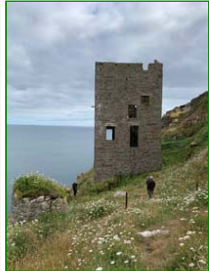
Members heading for the 1834 Old Engine shaft, Trewavas. (Gareth)
