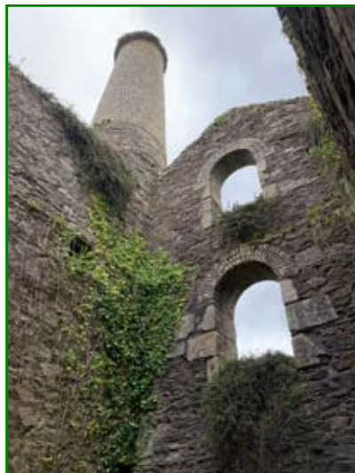
Interior rear wall of the stamps engine house. (Gareth Rushton)
