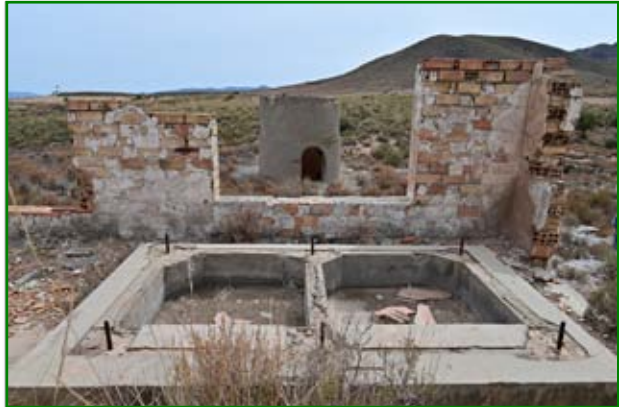
Engine foundations for a small electric winder by the shaft with the tall concrete surround. (Kelvin Lake)
