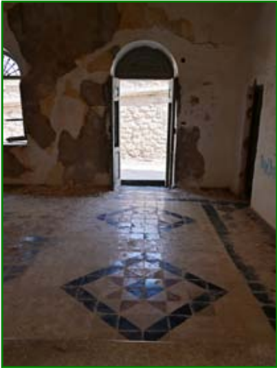
Interior of the stores building.
