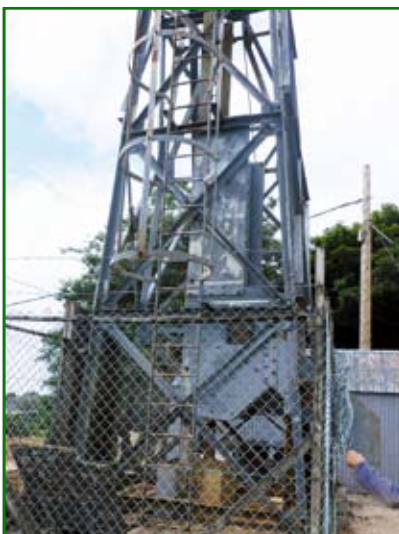
Vivian's shaft headgear, worked by the electric hoist. (Julian Bromhead)
