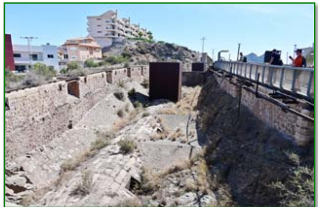
50,000 ton capacity iron ore hopper for Tunnel No.1.
