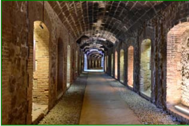
The renovated ore hopper tunnel, part of the museum.
