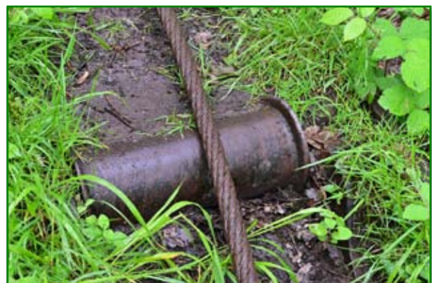
Cable and roller bearing on the A3 Garrett Incline.
