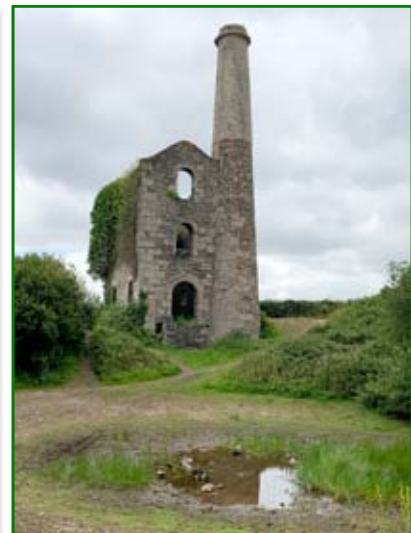
Rear of the engine house, with dried up engine pool in foreground.
