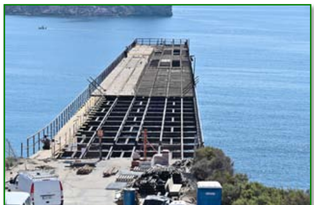
Restoration work underway on the pier decking.
