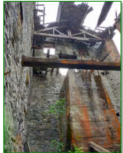
Interior of Klondyke mill. (Andy Wood)
