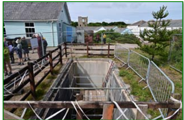
The newly re-constructed 'Sump' shaft. (Kelvin Lake)
