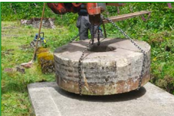
Putting the bedstone in place. (Andy Wood)
