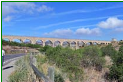
View of the aqueduct from the road.
