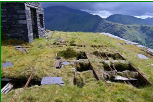
C6 Incline top, the drums are under the rails.
