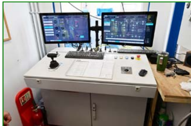
View from the winding driver's seat - there are 2 more monitors above those in the picture. (Kelvin Lake)
