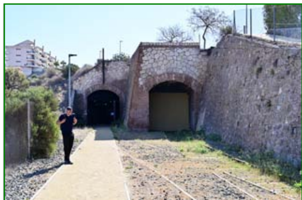
Entrance to the discharge tunnels for the ore hoppers.
