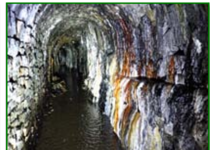
Stone lined level in Rampgill. (Vicky Robinson)
