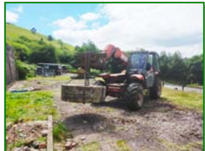
Moving the large bedstone to the plinth. (Andy Wood)
