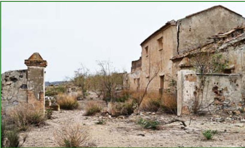
Entrance to the enclosed remains of the Sulphur Works.
