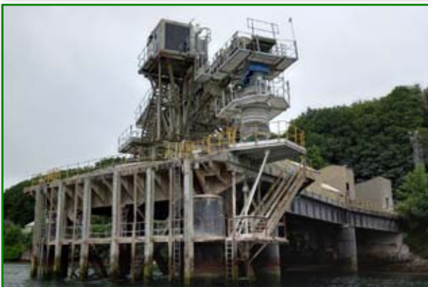
Detail of the ship loading facility. (Roger Gosling)
