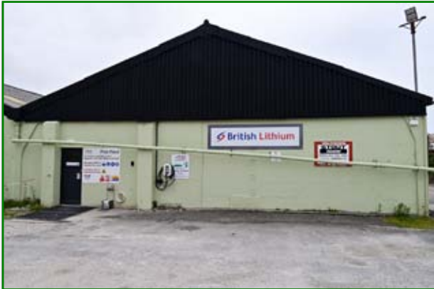
The Imerys British Lithium Pilot plant building.
