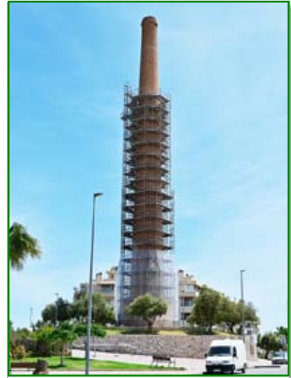
The La Loma smelter chimney.
