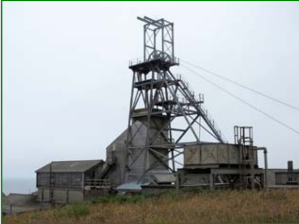
Headframe of the 480m deep Victory Shaft. (Graham Smith)
