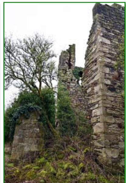
Remains of a chimney turret on the North-east corner of the building.
