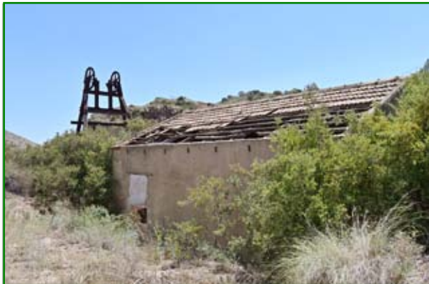
Mina Dios te ampare engine house and headframe.
