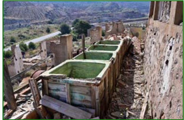
The row of 4 wooden tanks stained pale green (on the level above the ball mills. What caused the green stains? )
