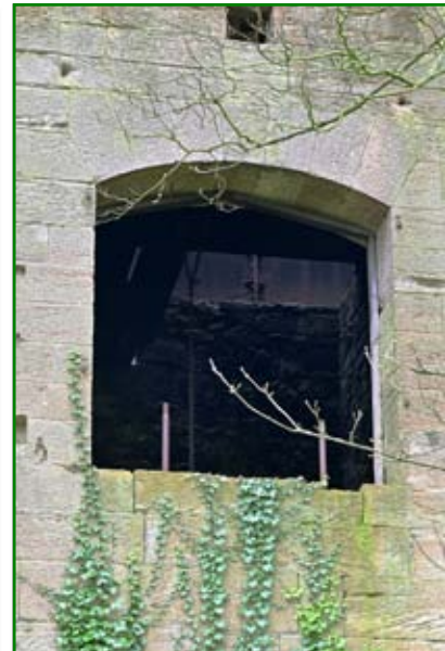
Detail of the bob wall and bolts on the water tower.
