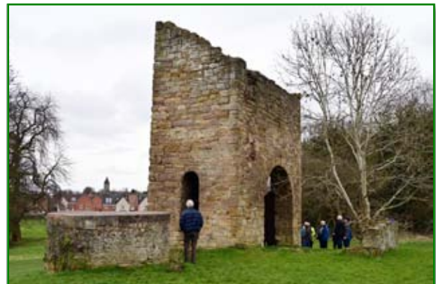
Bob wall and capped shaft (left) of the Kinningars Park engine house.
