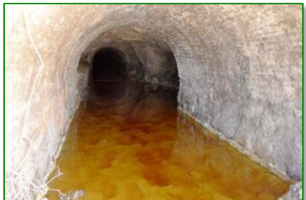
View into the tunnel.
