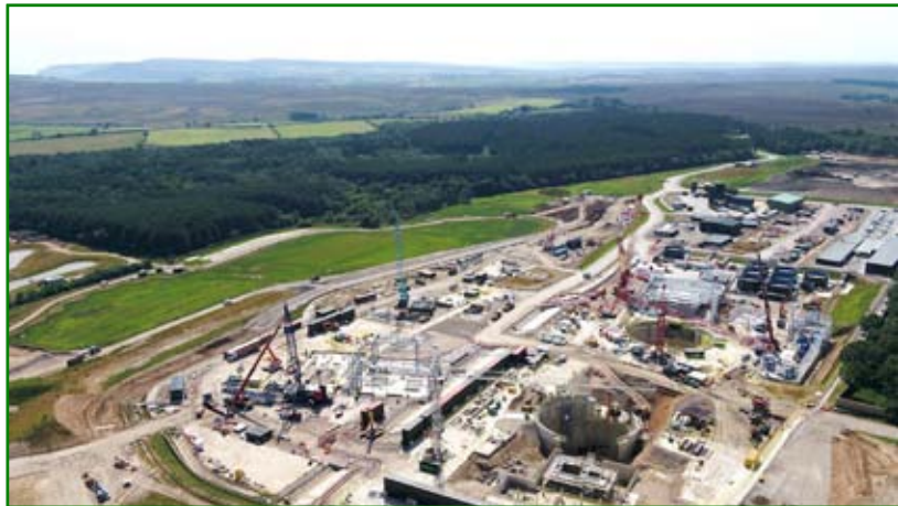
Woodsmith Mine aerial view, August 2019.
