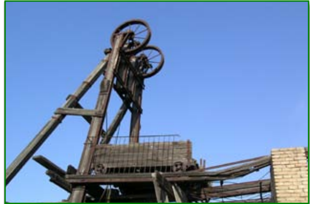
The shaft top arrangement at Mina San Simón. (2008)
