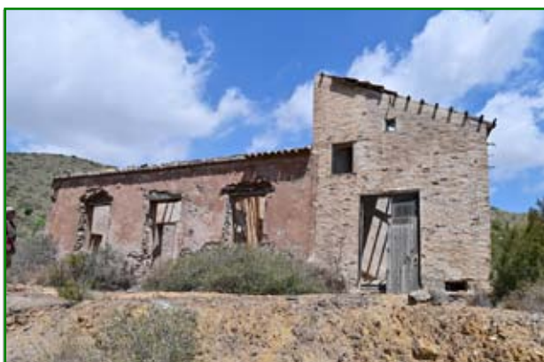
Office building at Mina Observacion a Santervas.
