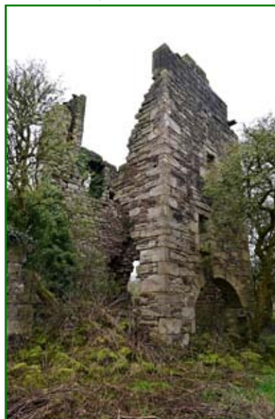
Blacksyke Engine House, built 1781. Note the boiler/cylinder arch.
