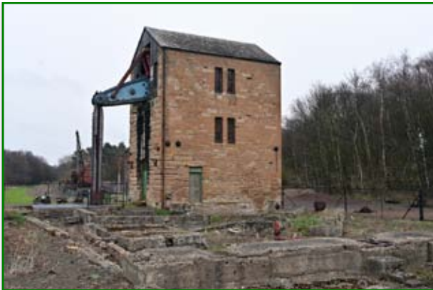
The Category A listed pumping engine house, complete with its Cornish beam pumping engine.
