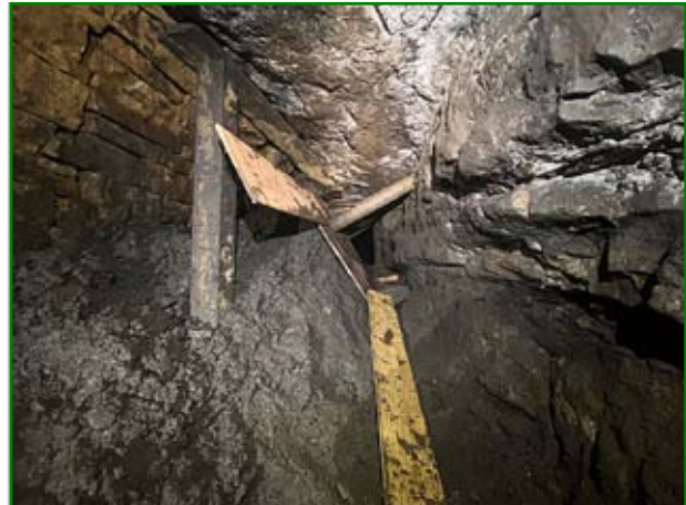
Temporary shoring put in after escape. (Matt Clarke)
