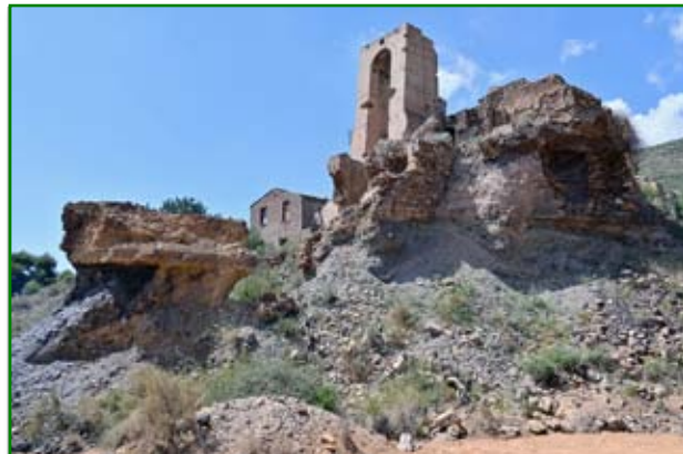
Masonry headframe and engine house, Mina Inocente.
