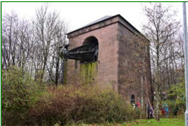
The Devon Colliery Cornish beam pumping engine house with its cast iron beam and pump rod.
