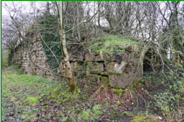
Twin lime kilns near the Blacksyke Engine House of Caprington Colliery. (Kelvin Lake)
