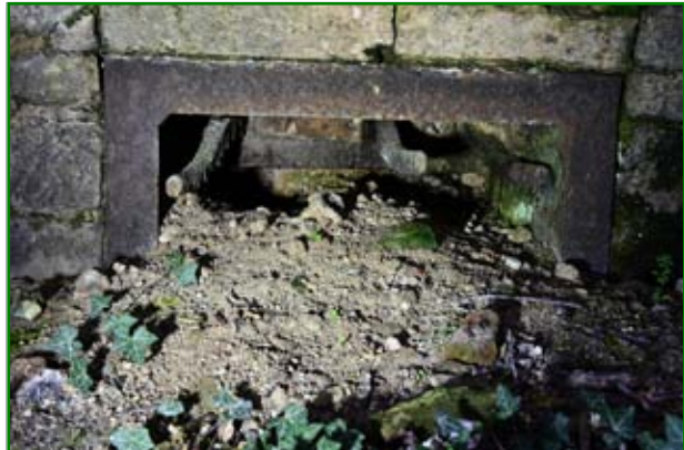
The grate of one of the lime kilns, complete with bars.
