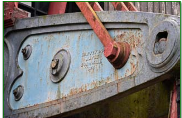
The cast iron beam made by Harvey & Co of Hayle in 1874.
