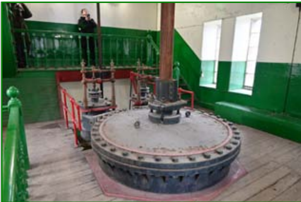
Top of the 70" diameter cylinder of the Category A listed Cornish beam pump.
