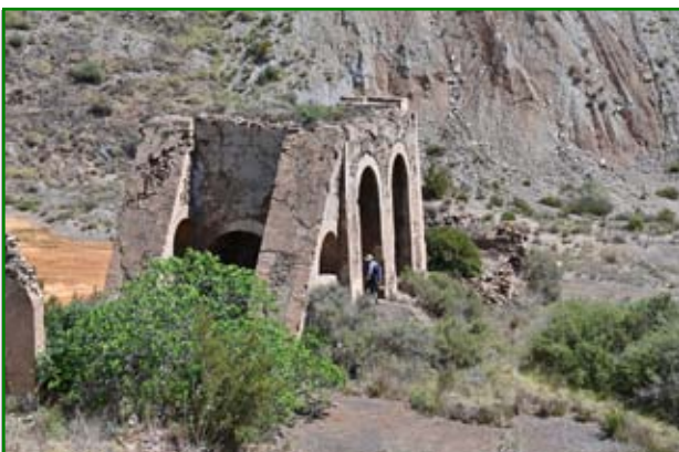
Julian by the Masonry headframe block, Mina Inocente.
