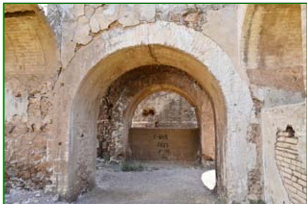
Shaft under the masonry headframe at Mina Inocente.
