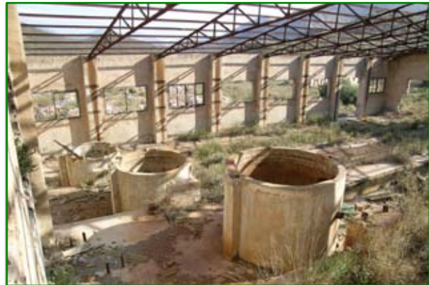
Flotation cell area with roof girders in 2008.
