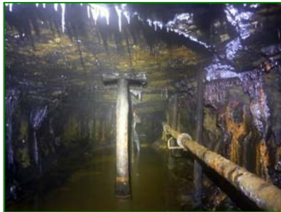
Following the compressor pipe. (Julian Bromhead)
