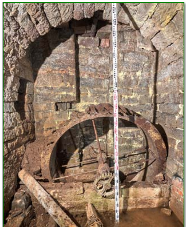
The 1.85m diameter overshot waterwheel in the chamber off the main line of the tunnel. Water for the wheel came in from the void middle left - possibly via the large loose iron pipe lying bottom left of the picture. (Ian Cooper)
