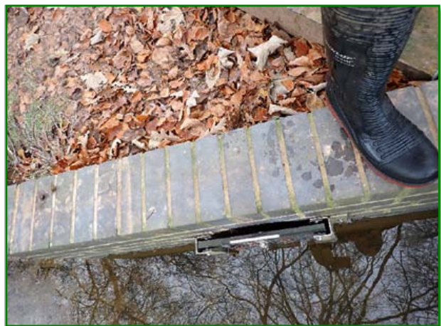
2. Looking down at the gate to the pool.
