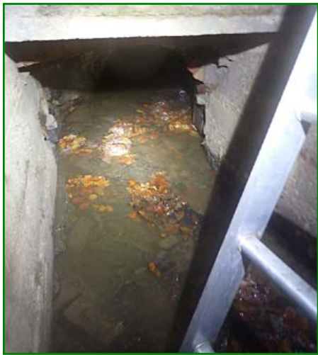
5. View below the manhole. (Steve Holding)
