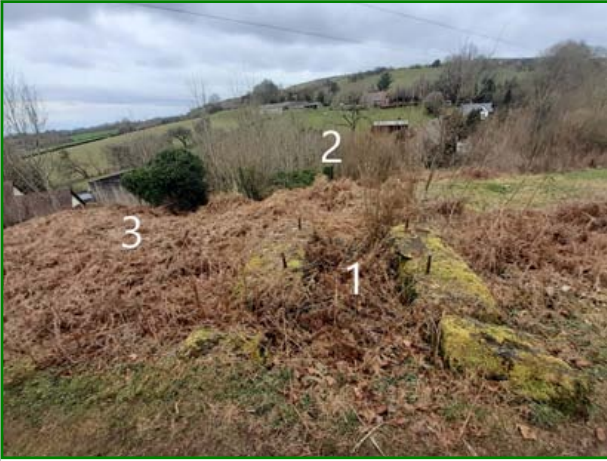
Figure 7: Crusher plant, looking north. In the foreground are machine bases (1), behind are the tops of the pylons (2) and to the left is the tank (3). (David Poyner)
