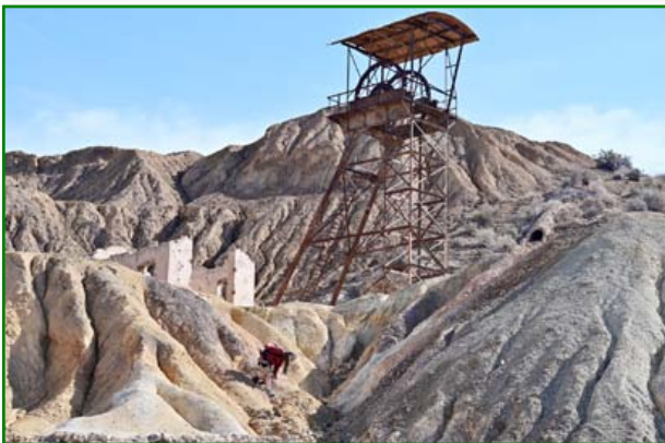
Headgear at Mina No Te Escapara. Two of the sheaves have been converted to use round rope. (Kelvin Lake)
