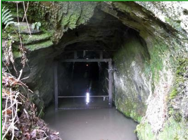
Deep Adit entrance.
