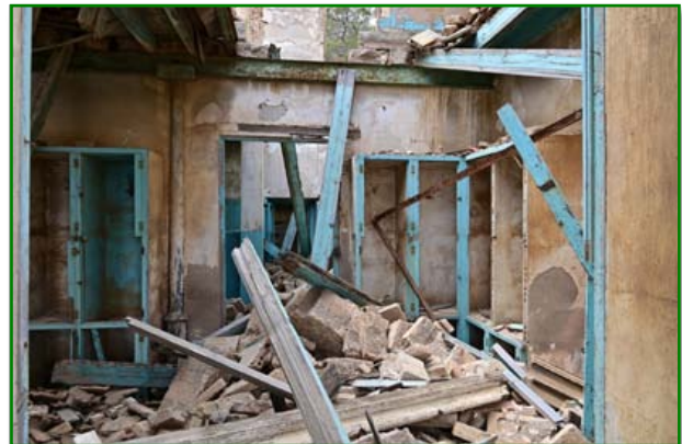
The Mina San Isidoro locker room near the Mina Iberia winding engine house. (Kelvin Lake)
