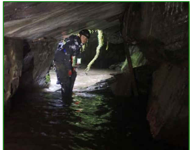
Emily in the main drainage level just before it enters one of the open quarry pits. (Graham Smith)
