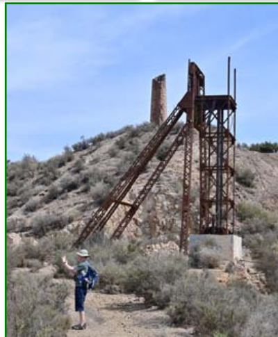
Julian by the headframe of Mina San Antonio de Padua with 2 cages
