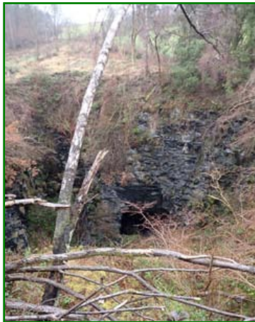
View down the overgrown incline. (Graham Smith)
