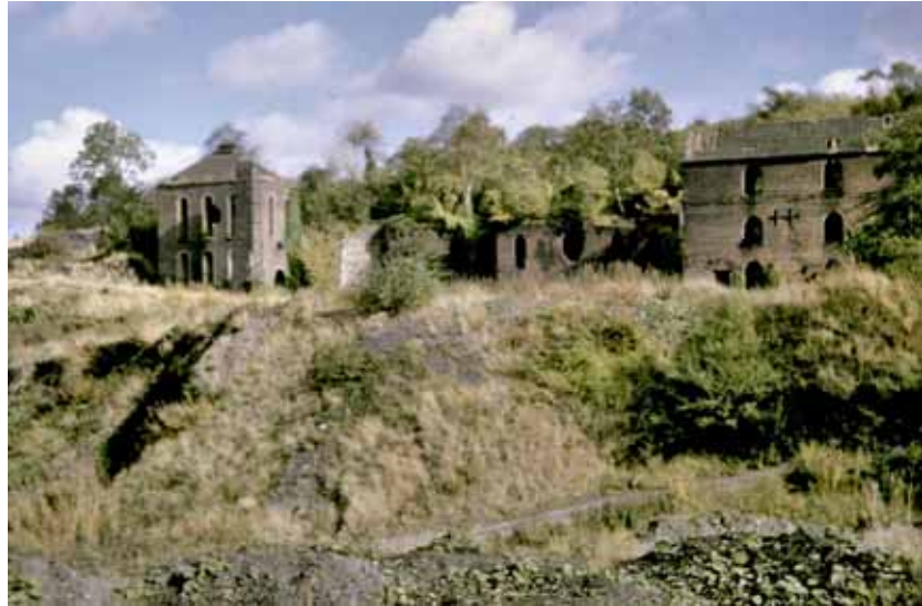
Slag Removal at Blists Hill Furnaces, October 1964.
