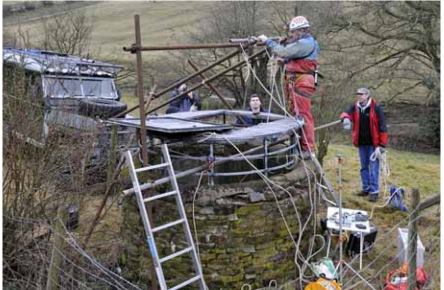
Above: Rigging the temporary inspection headframe on Chapel shaft.
