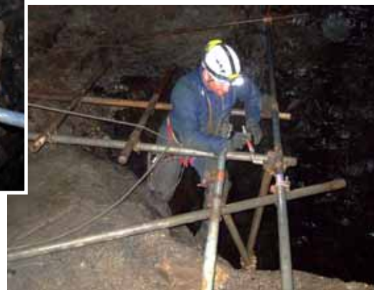
Below: Anchor points on one side of the platform, utilising original wall pockets, but with additional safety chains. (Andy Kennelly)
