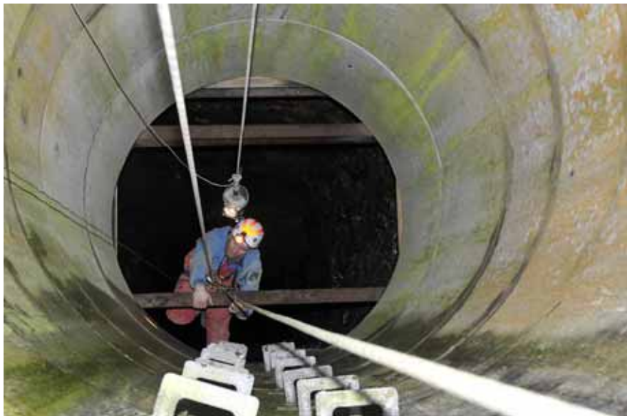
Below: Anchor points on one side of the platform, utilising original wall pockets, but with additional safety chains. (Andy Kennelly)
