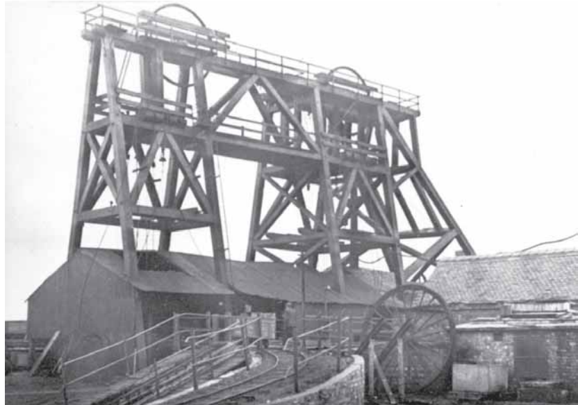
Photograph 2: Kemberton Pit c1945 showing the substantial timber tandem headframe built after the 1912 expansion. (Ivor Brown)
