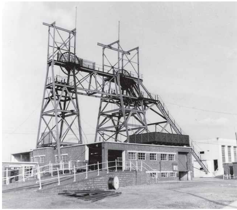
Photograph 2: Kemberton Pit c1945 showing the substantial timber tandem headframe built after the 1912 expansion. (Ivor Brown)
