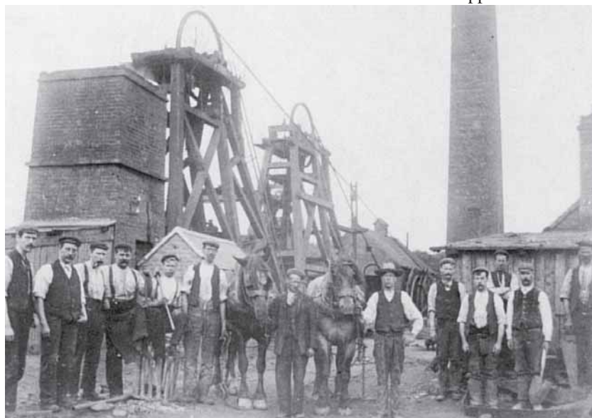
Photograph 1: Kemberton Pit c1900 with separate wooden headframes over each shaft. (Frank Turner)
