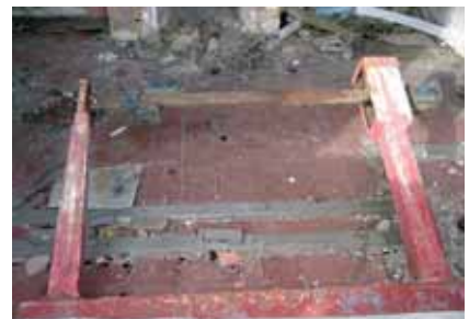
Figure 8: Steelyard inside the Alveley weighbridge; this has been pushed over and is now lying on the floor.
