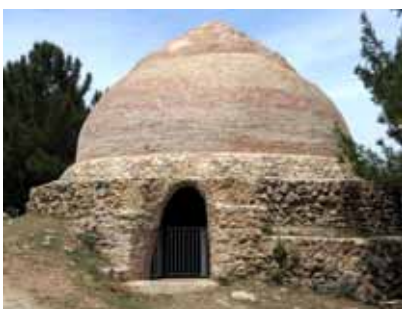
Above: A pozo complete with domed roof.
