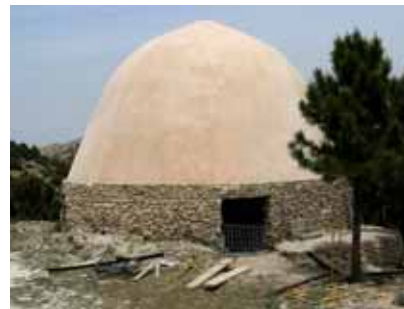
Above: Restoration in progress on another pozo.
