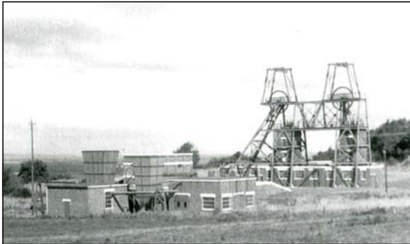
Figure 3 Methane extraction plant alongside main fan buildings at Grange Pit, 1960s
