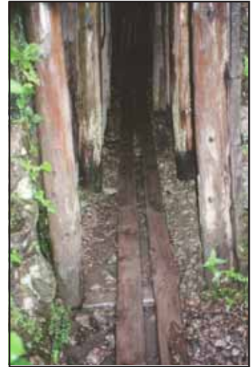
Above: Reconstructed mine timber work, including 'rails' in the entrance to "Die Aych" a mine dating from 1560, now the exit of the St. Louis Eisenthür Mine tour run by ASEPM.
