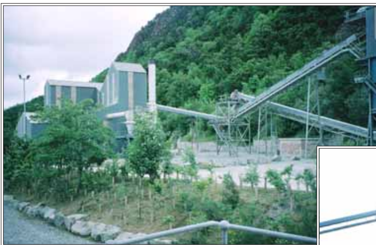
Left and Below: Main processing plant, conveyors and storage hoppers with loading bays for the graded rock.
