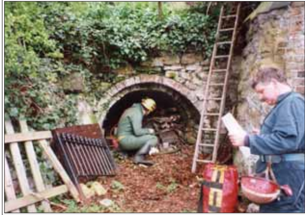
Above: Opening up the mine entrance
