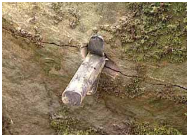
After a few hits with the hammer, the rock begins to split along a line joining the holes.
