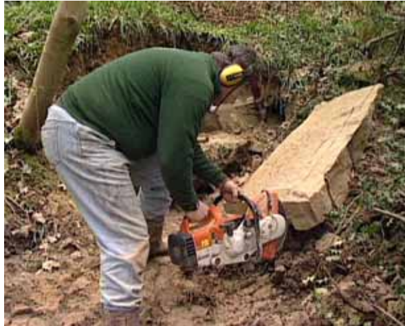
Cutting the stone roughly to shape using a disc cutter
