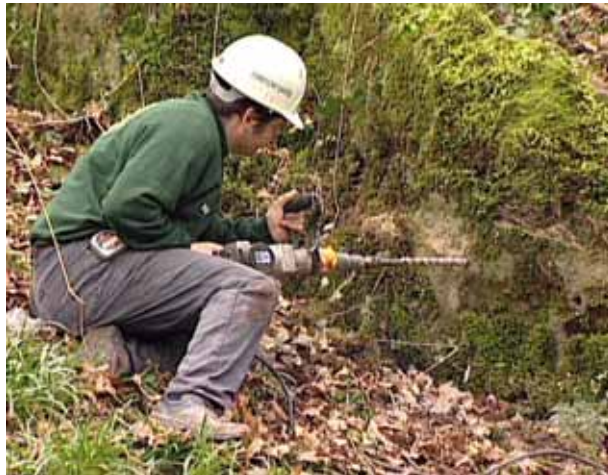
Drilling the holes for the plug and feathers
