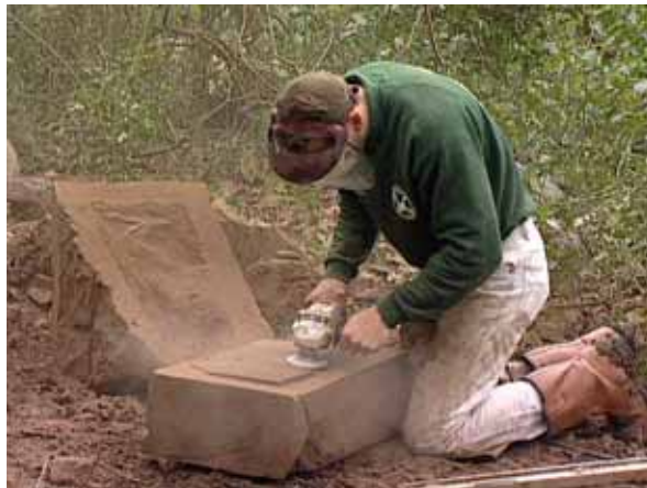
Shaping the stone with an angle grinder. Final polishing was done later.
