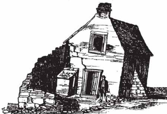
A sketch of housing (c1843) that accompanied the report, to illustrate the affects of subsidence on the area.
