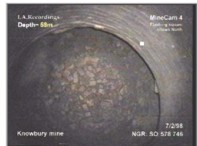
Base of shaft, showing blockage and end of brickwork.
