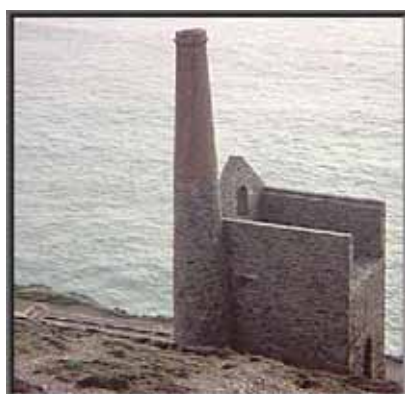
Above: Towanroath Pumping Engine House, with later horizontal engine bed on the left.
