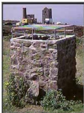
Preserved and gridded shaft at Wheal Coates, Stamps and Whim Engine houses in background
