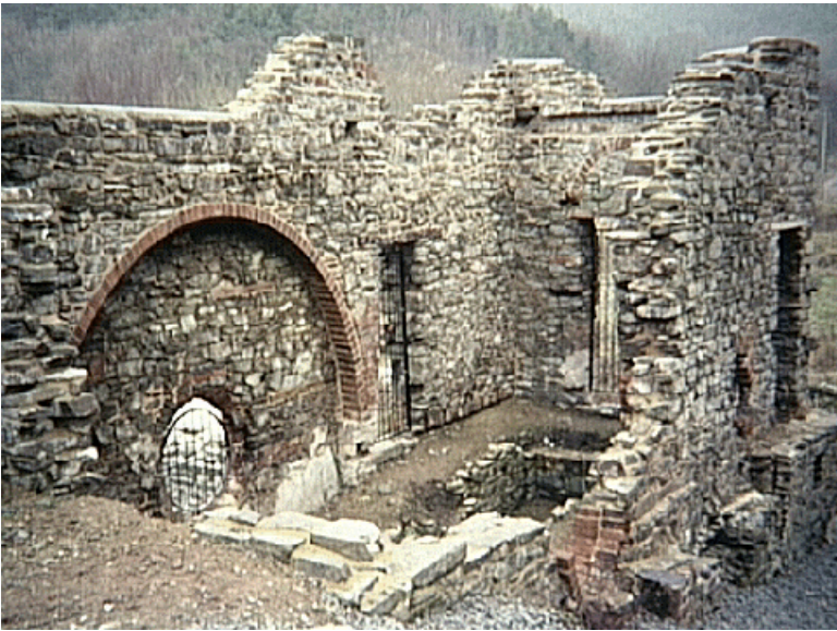
Above: The 'exposed' New Crusher house at Snailbeach
