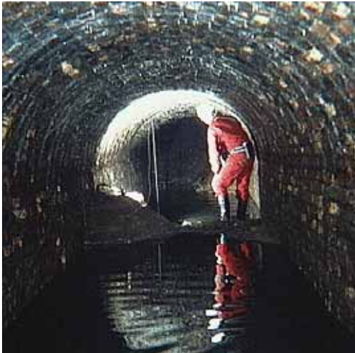
Right: Inside the 'tramway' tunnel near the top of the 'Wynd', Cherry Tree Hill, Coalbrookdale (looking in the direction of the top of the incline).
