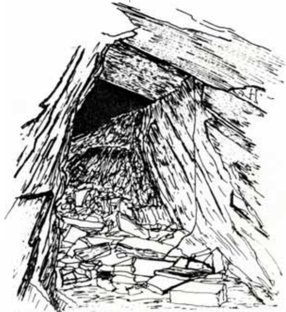
COLLAPSED WALL IN CHAMBER 1 EAST BACK VEIN FLOOR E, CWMORTHIN
