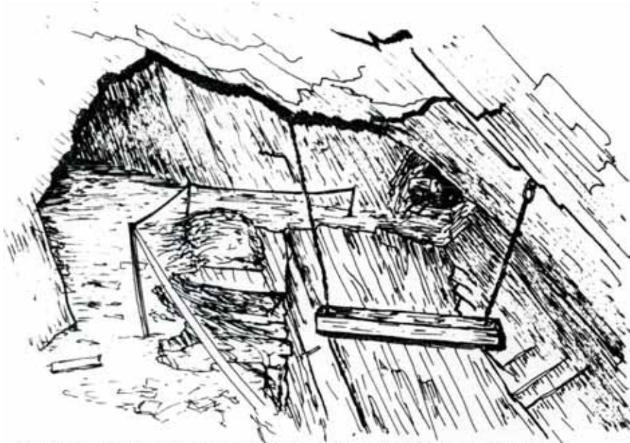
REMAINS OF BRIDGE IN CHAMBER 2 WEST FLOOR D CWMORTHIN
